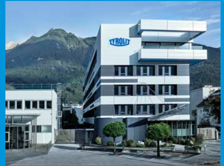
TYROLIT headquarters in Schwaz (Austria)
